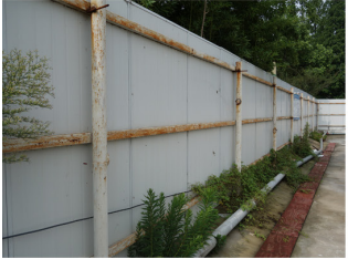
THE WALL HERE
